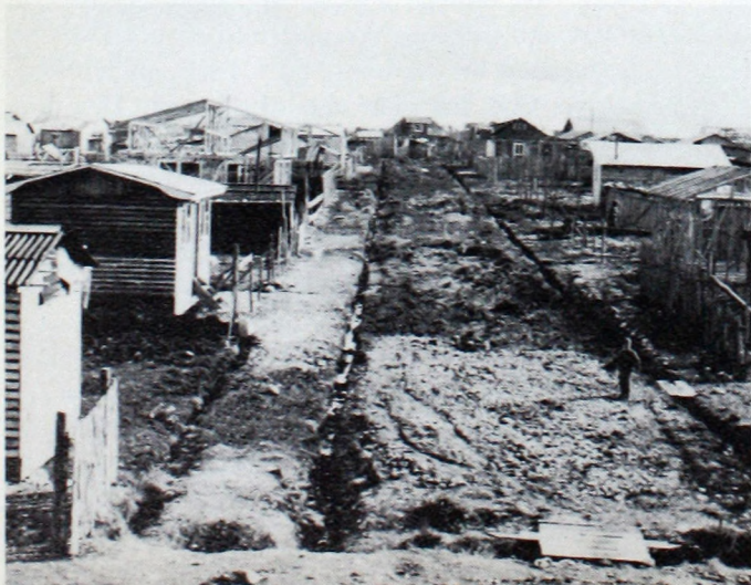
A typical self-help housing project includes building a street.
